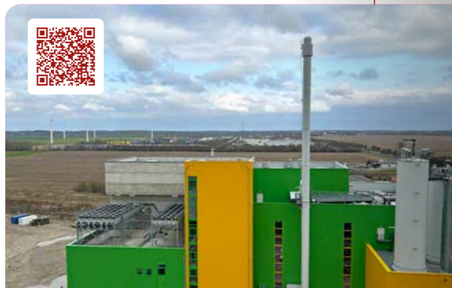
Transforming waste into a resource: The sewage sludge mono-incineration plant in Stavenhagen will start regular operations as of 2024 and supply district heating for the city.
