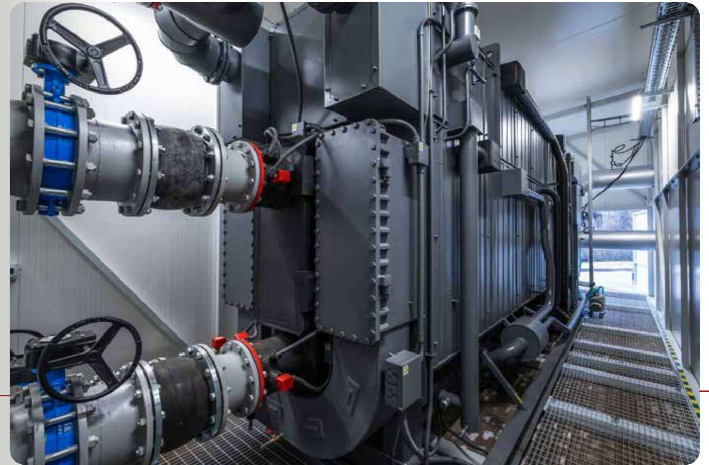
Innovative technology: an absorption heat pump - a step towards decarbonising the heat supply
